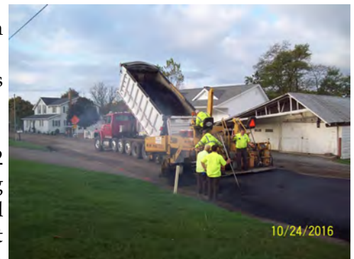
County Road 10 FDR with asphalt
