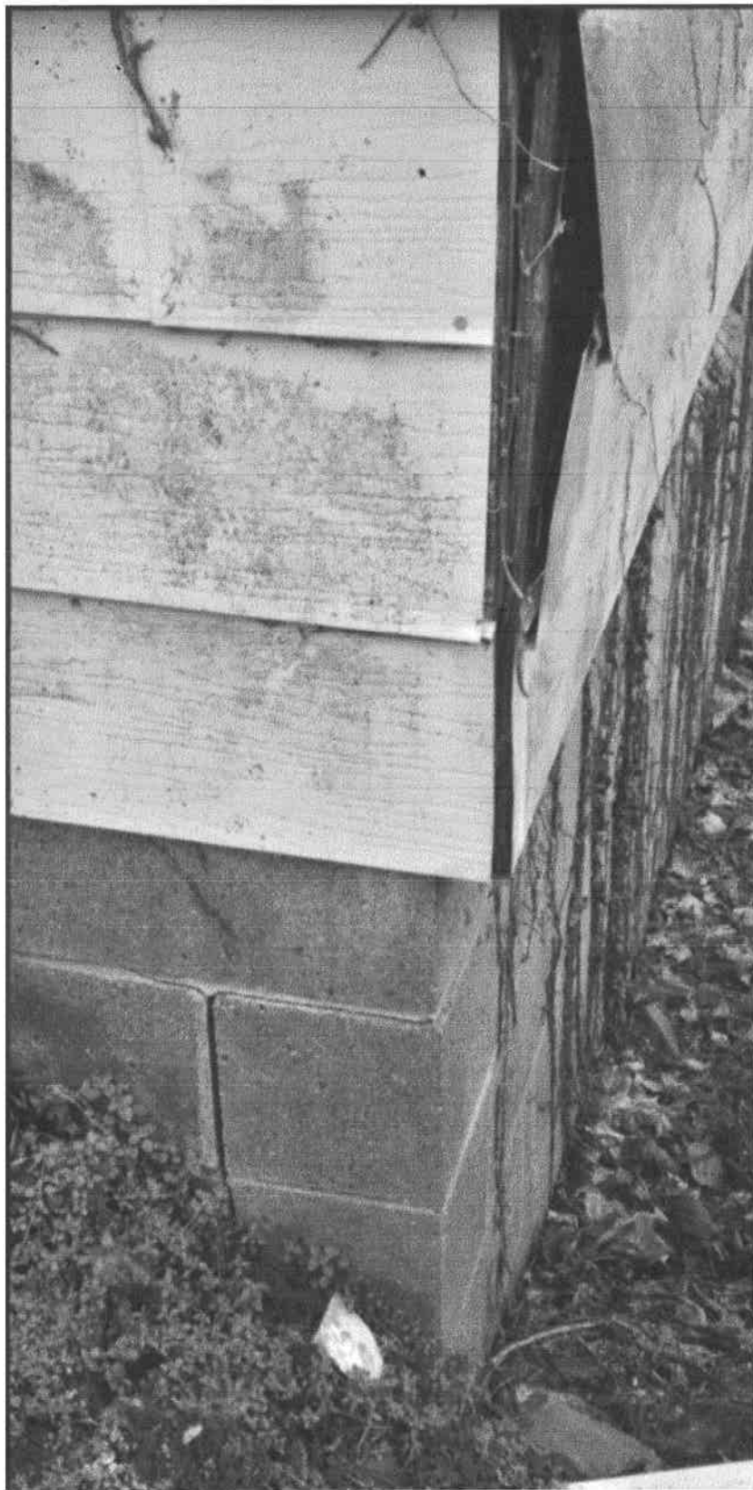
Corner siding + foundation damage + plant growth
