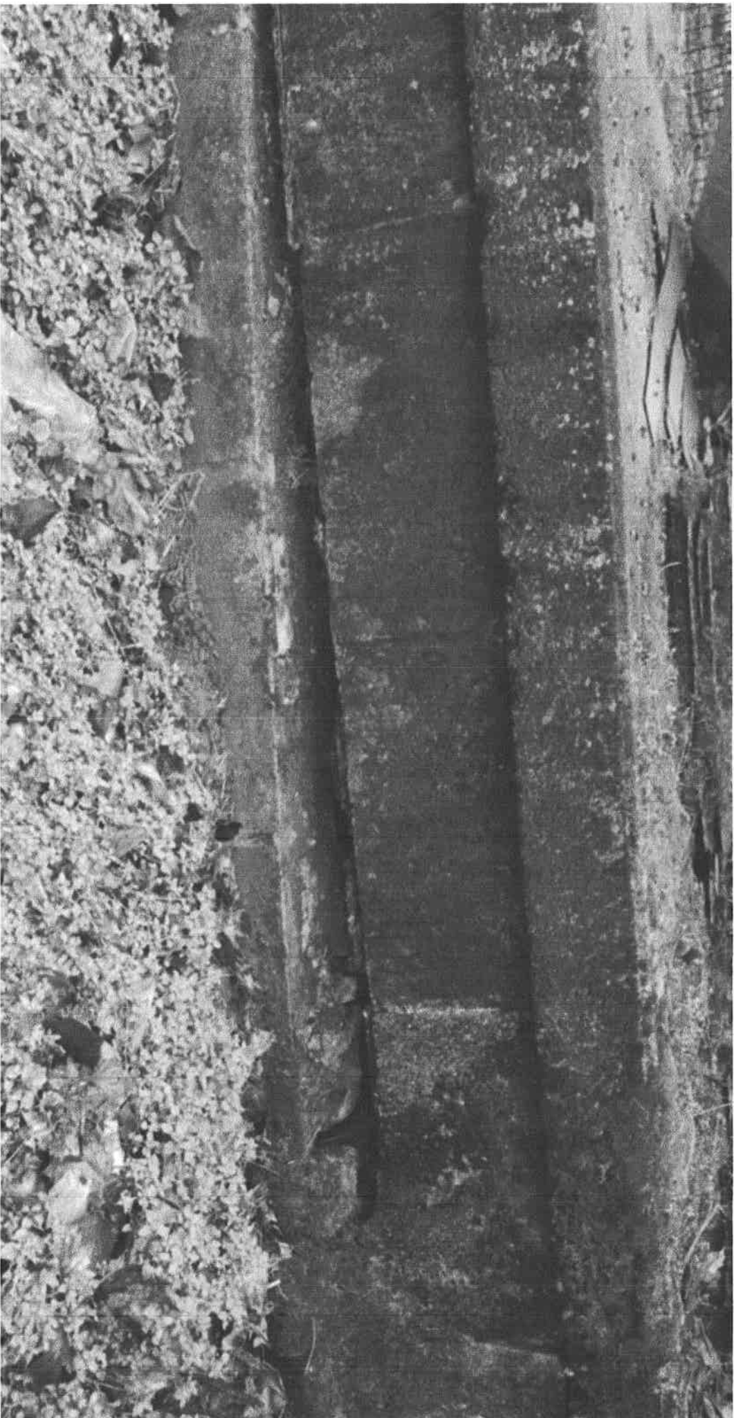
Front masonry stoop sinking + separating
